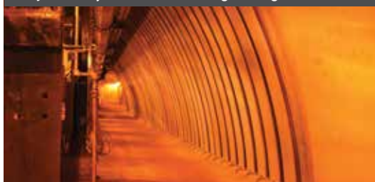
Roy Hill Project - Tunnel Strengthening Works
