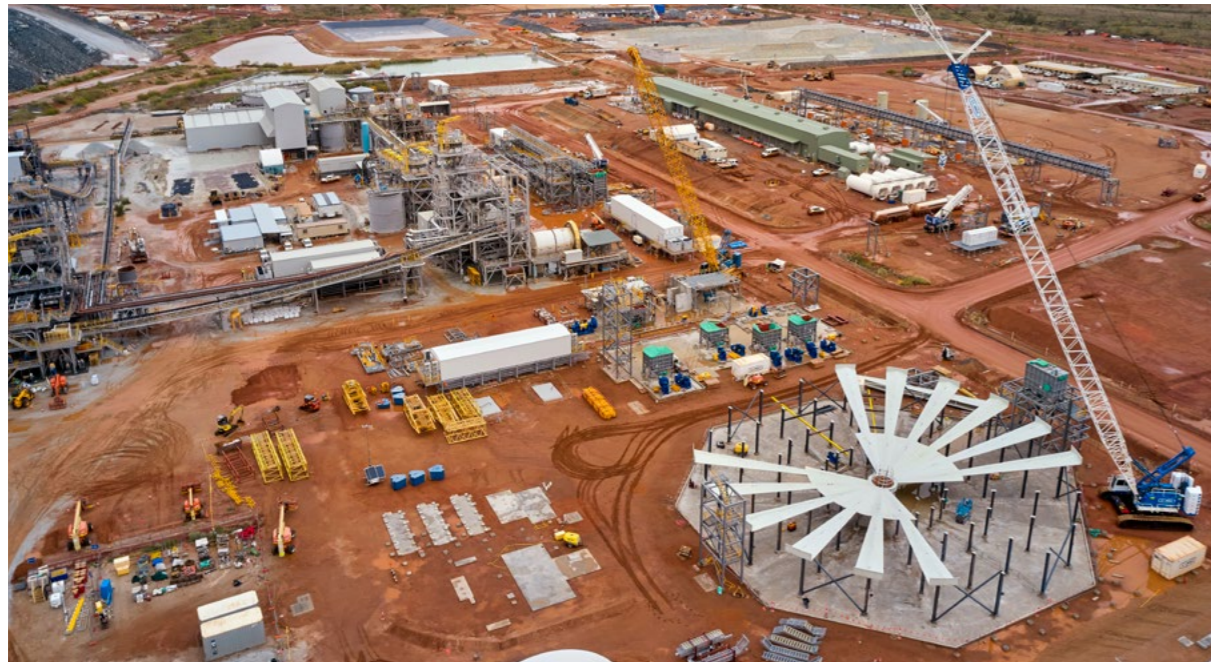
Pilbara Minerals' P1000 Expansion Project, June 2024
